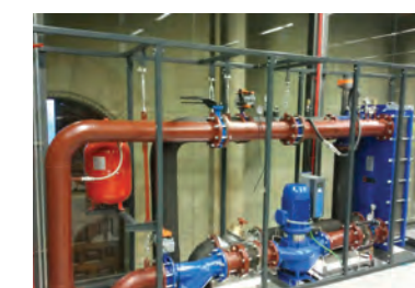
Chill Water Exchanger
