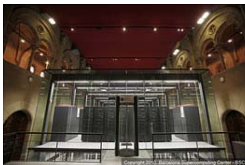
Barcelona Supercomputing Center
